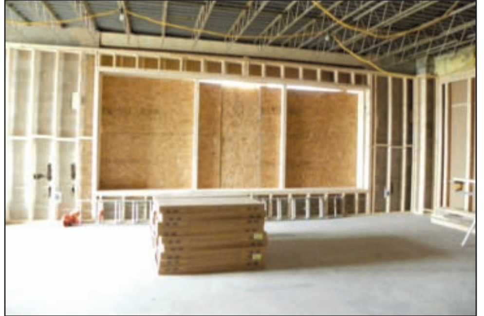
Renovations are underway for the Window and Door Showroom. (Thompson photo)
